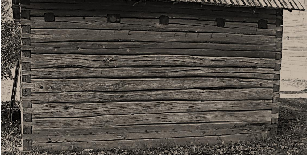
Figure 5.2 Dovetailed Broad Axe Hewn Construction. (Photo by Author)
