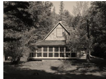
Figure 5.6 Sevona Memorial Cottage. (Photo by Author)
